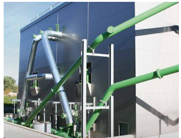
Discharge system of a Kompogas® concrete digester
